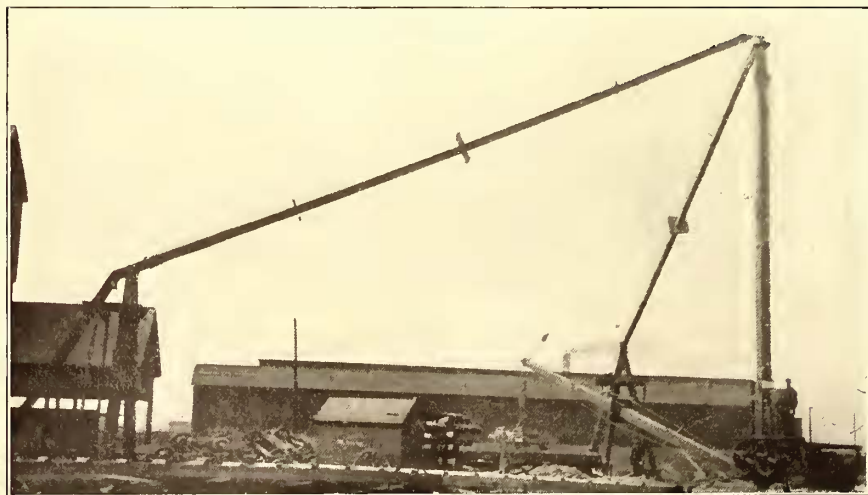
THE MOTOR-DRIVEN DERRICK AT WORK IN THE YARDS OF THE DETROIT UNITED RAILWAY
