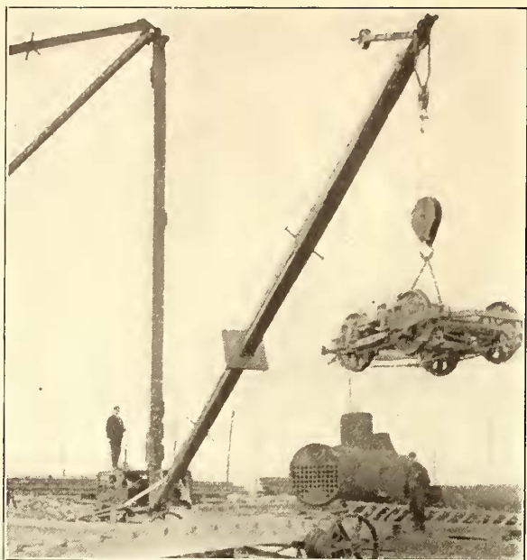
MOTOR-DRIVEN DERRICK LIFTING CAR TRUCK
